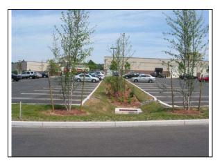
Figure 5-9. Typical Concave Bioretention System
